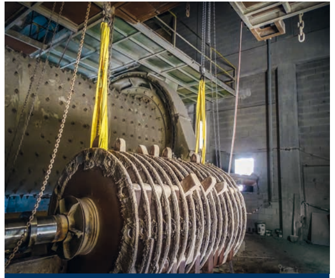
Lifting operation using round slings
