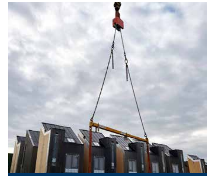
Levo load balancer use to install sloped roof systems
